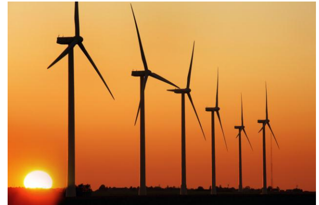
Alstom 2010. Photo courtesy of DOE/NREL
