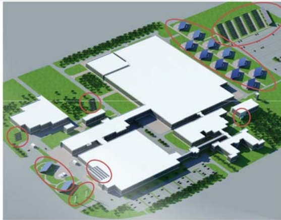
Energy Solutions Park, Bielefeld, Germany
