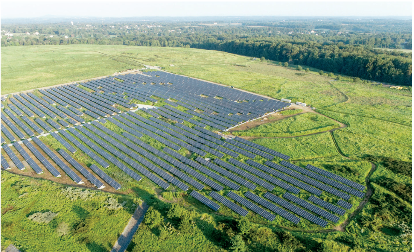
MEA Community Solar LMI-PPA-funded Oaks Landfill Community Solar Array's aerial view. Photo: Maryland Energy Administration
