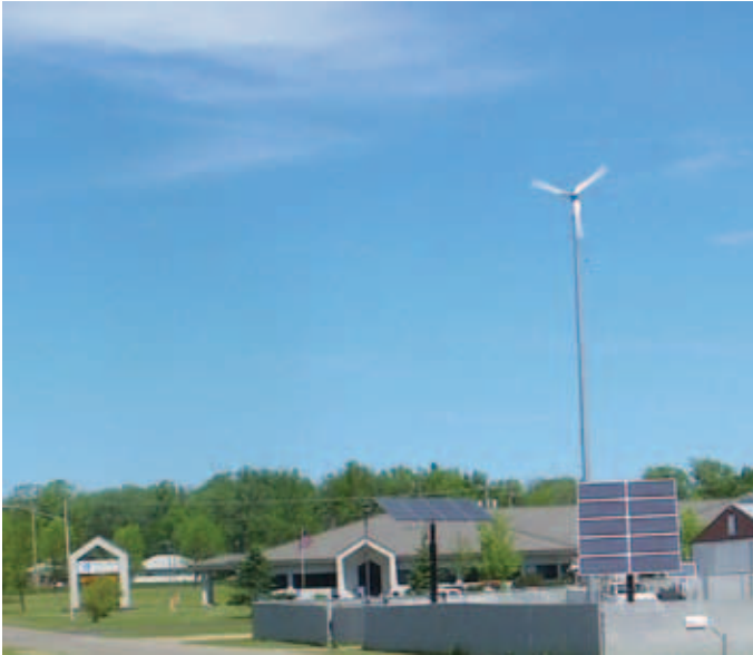
Xcel Energy's Renewable Development Fund's Renewable Energy Kit for Remote Telecom Equipment
