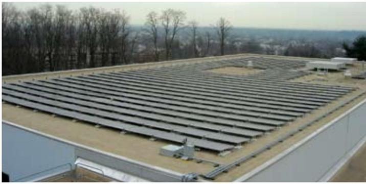
Ortho McNeil Pharmaceutical, a Johnson & Johnson company, installed a 510-kilowatt solar electric system at its campus in Raritan. The installation produces enough electricity to power about 45 average homes.
