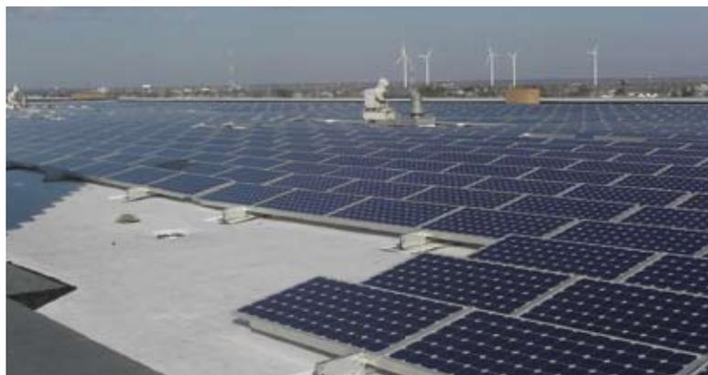
The Atlantic City Convention Center is one of the largest roof-mounted solar PV systems in North America, rated at 2.36MW of dc capacity. Higher valued SRECs enable profitable investments in solar without large rebates.
