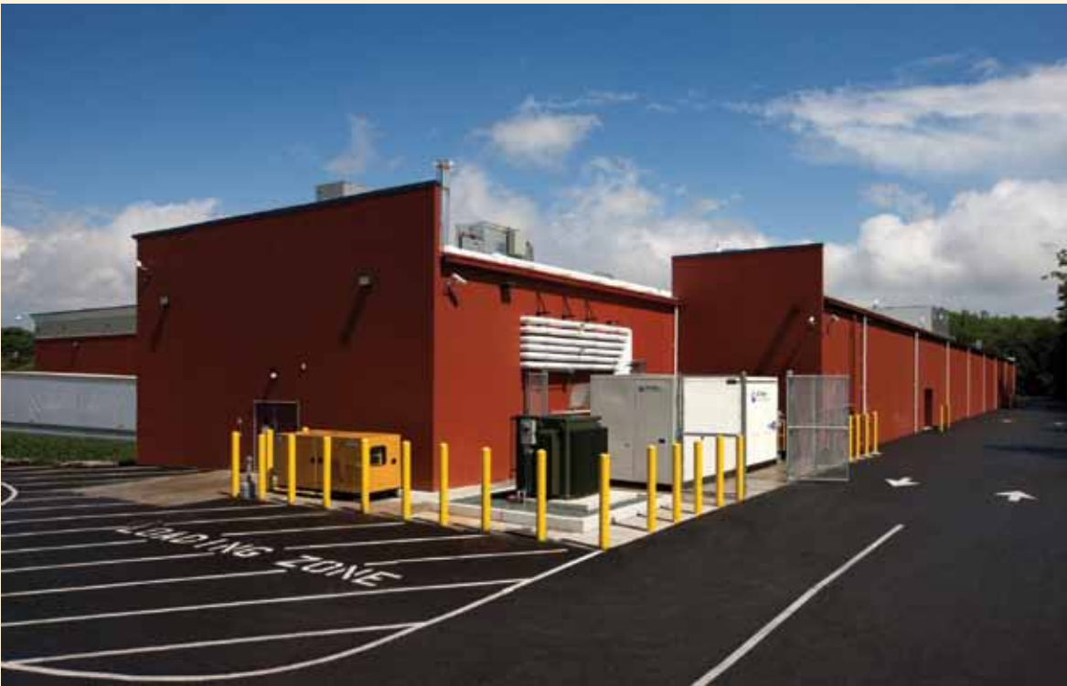
Price Chopper's first fuel cell installation in Colonie, New York.
