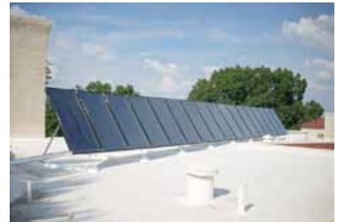
SDF provided a modest grant to Rushforth Solar, Inc. to help reduce the sale cost of four solar domestic hot water systems in apartment buildings in the Philadelphia area. The key to these cost-effective solar installations for commercial buildings with centrally heated hot water is the hot water storage tank, which is at atmospheric pressure and can be assembled on-site at a low cost.
