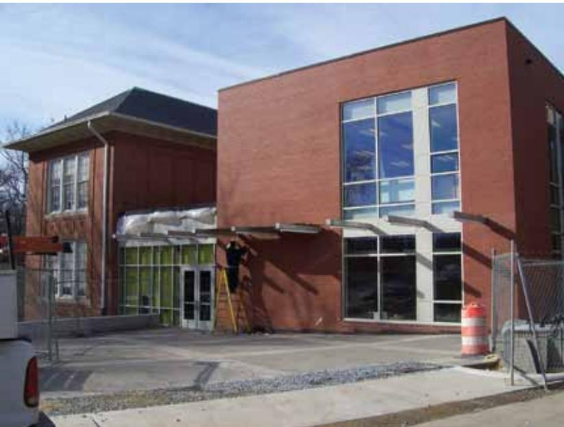
TRF Energy financed the energy retrofit of existing space and an energy-efficient addition at the Latin American Montessori Bilingual Public Charter School in Washington, D.C. The energy measures included a high-efficiency modular boiler heating system, a high-performance building envelope with daylighting features, energy-efficient lighting fixtures and controls, and a green roof for capturing storm water.
