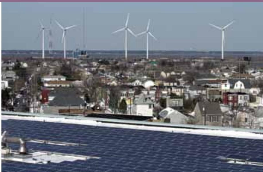
From the roof of the Atlantic City Convention Center, you can see both the Atlantic City Convention and Visitors Authority's 2.37 MW solar energy installation, the largest roof-mounted solar PV system in the U.S., and the Atlantic County Utilities Authority's five 1.5 MW wind turbines, the first utility-scale coastal wind installation in the eastern U.S.
