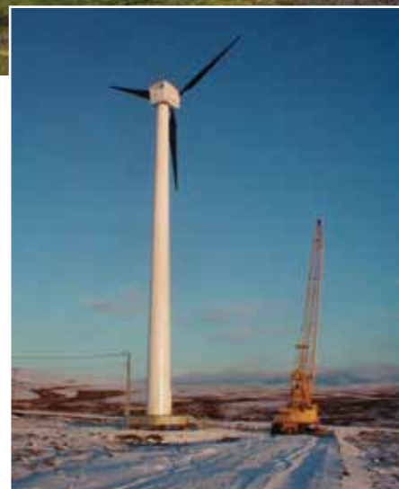
100 kW Northwind 100 Wind Turbine Installation, Toksook Bay
